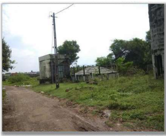
Figure No 42. Under Ground water Tank
