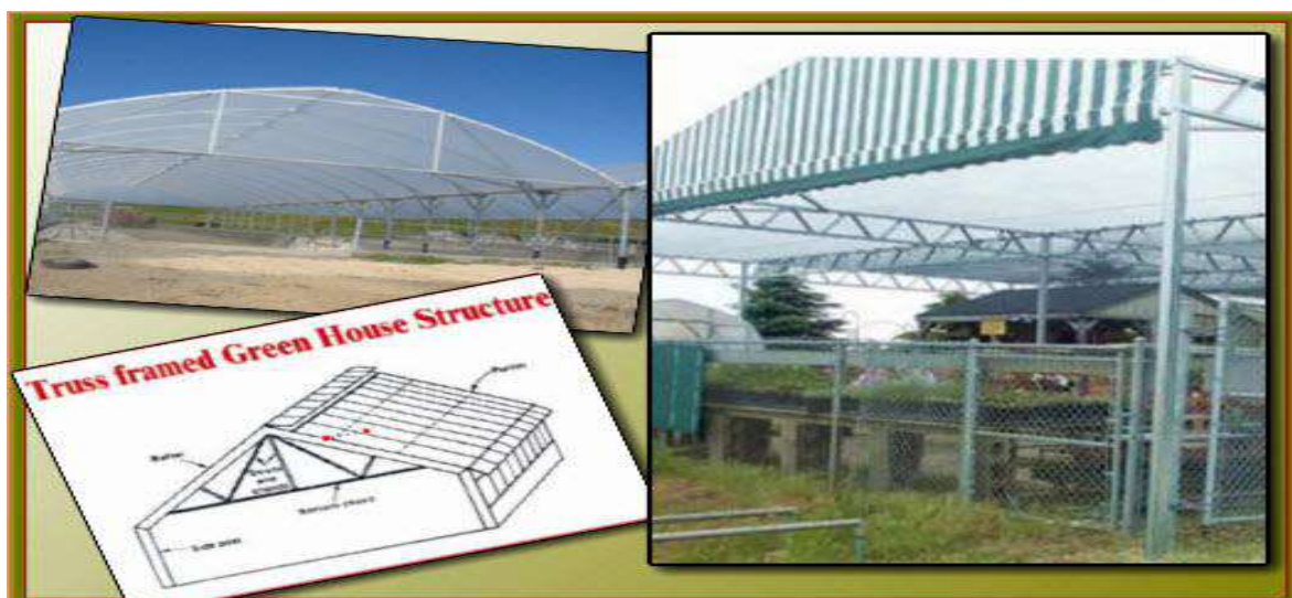
Figure No 129 truss framed green house structure
