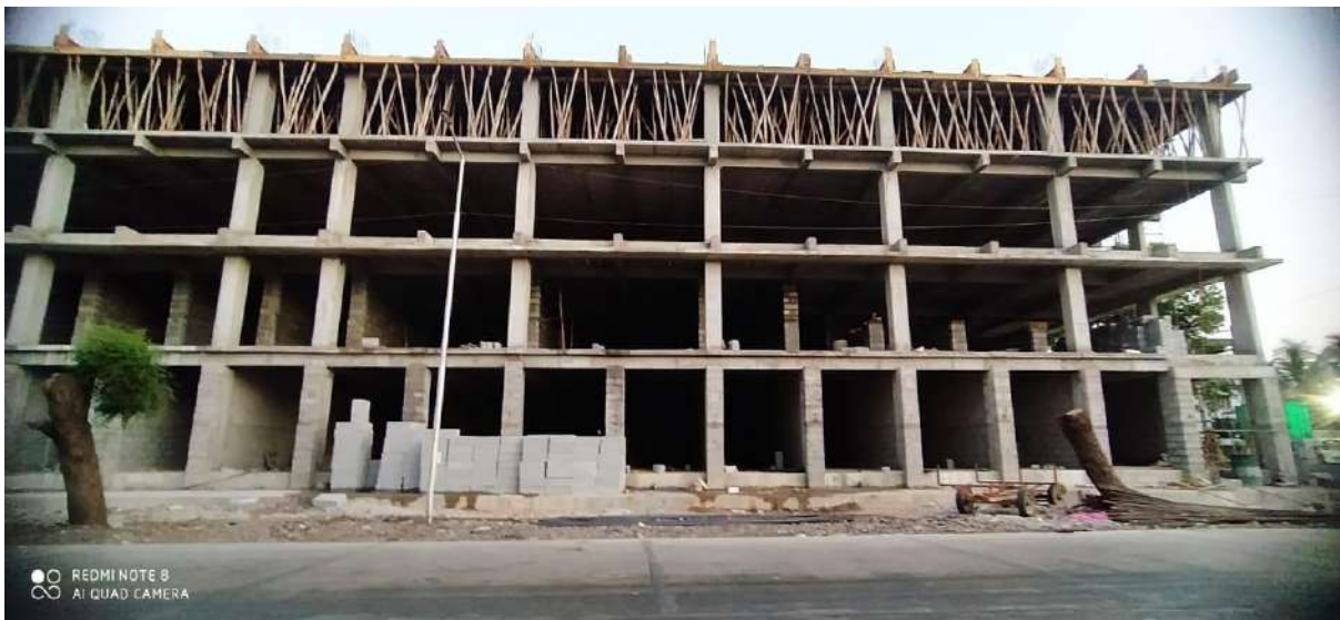
Figure No 115 photograph's during constructions work
