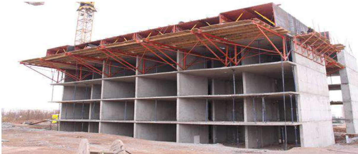
Figure No 101 Tunnel Formwork System
