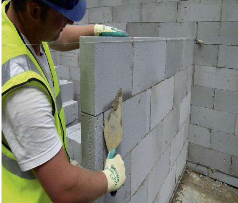
Figure No 103 Thin Joint Masonry Technique.
