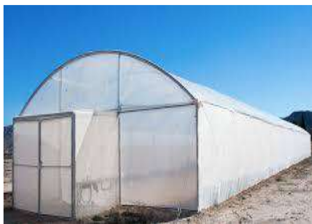
Figure NO 137 low cost green house
