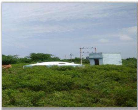
Figure No 39. Under Ground Slump
